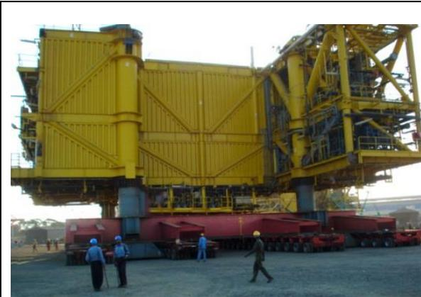
SPMT loadout of offshore structure
