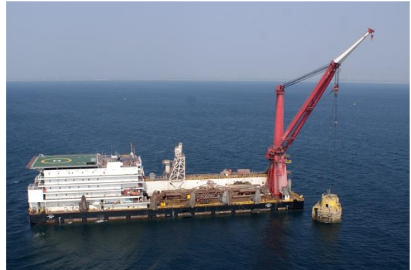
Salvage, refurbishment and reinstallation of SPM buoy
