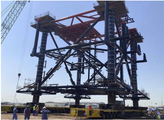
SPMT loadout of offshore structure
