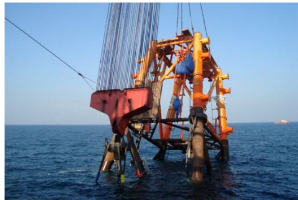
Heavy lift and installation of offshore structure of about 3000MT
